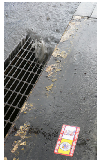
Figure 2. Runoff (Image source: City of Santa Fe Stormwater Management)
