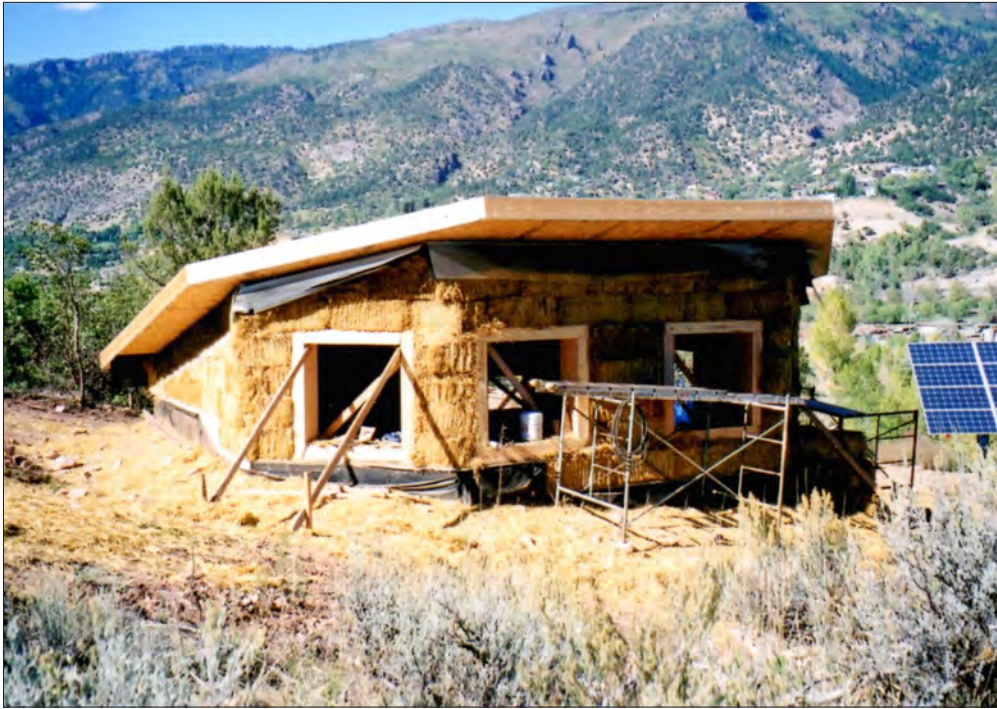
A student-built, strawbale classroom arises on the hillside campus of Yampah Mountain High School.
